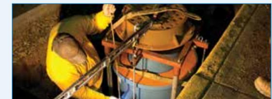
Failing Steel Interceptor Replaced with TZ-400 in Traffic Rated Zone Outside Fast-Casual Restaurant using One-Pour System
