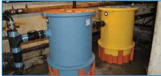
A Solids Separator installed ahead of a Trapzilla® GI servicing the food prep area of a national grocery chain.
