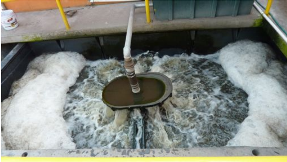
Figure 6 – Top View of A Bioreactor with MicroFast®
