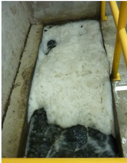
Figure 5 – Top View of A Bioreactor with Free Floating Biomass Carriers
