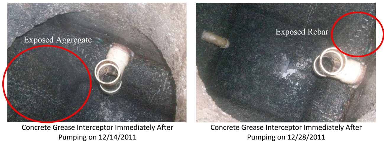
Figure 5-6, Concrete Grease Interceptor Observations
