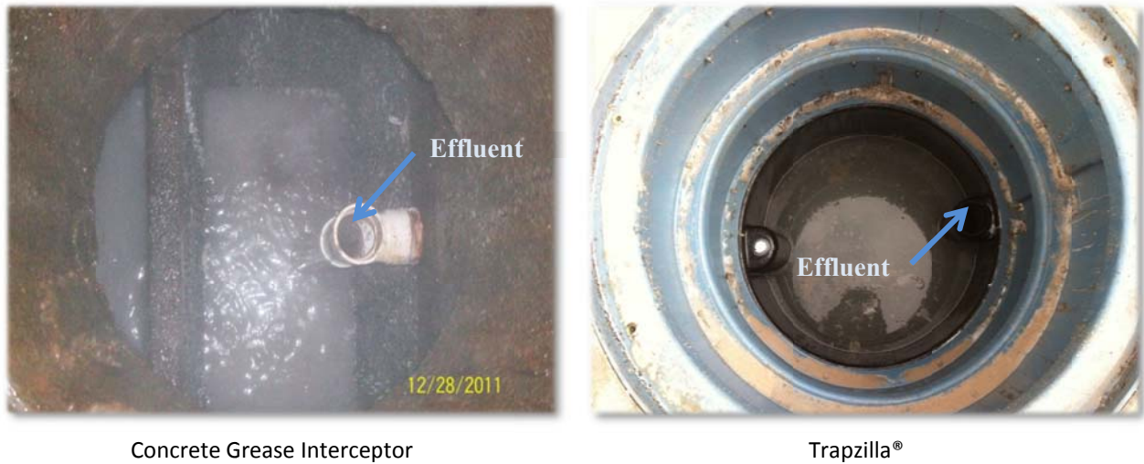
Figure 4-1, Effluent Sample Collection Points
